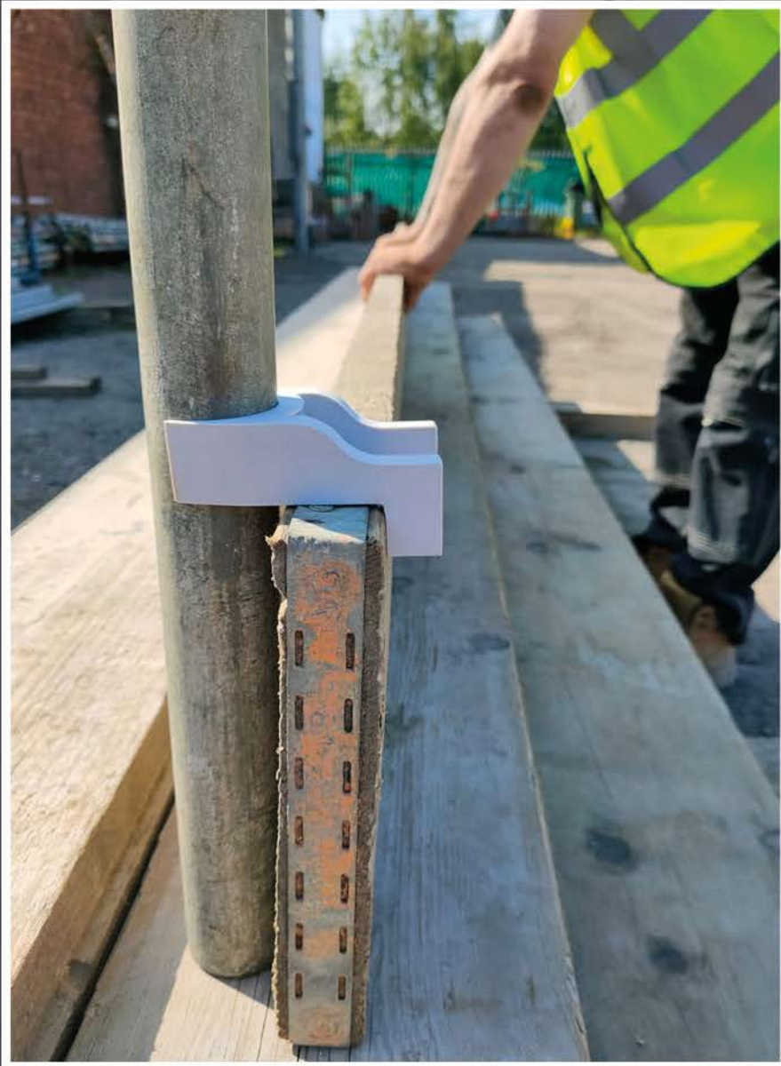
Edge toe board held in place with a toe board clip
